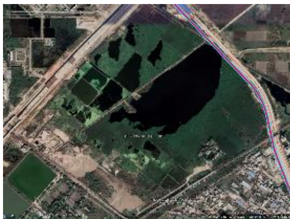
Figure A: Google Earth Image of February 2024 - Before Drainage Repair
