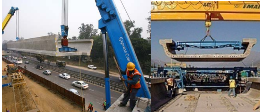
FIGURE 5.29: LAUNCHING OF U-CHANNEL GIRDER
