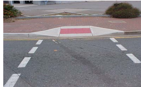
Ramp from footpath to carriageway for easy movement
