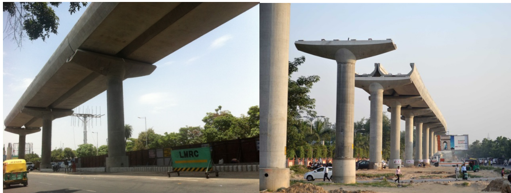
FIGURE 5.28: PRECAST U-CHANNEL SUPERSTRUCTURE
