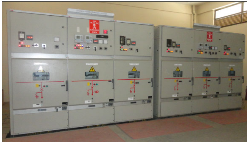
FIGURE 12.4: TYPICAL INDOOR AUXILIARY SUB-STATION
