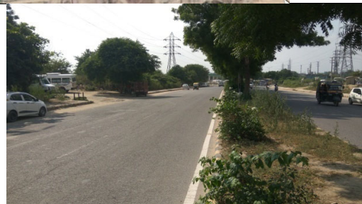
Station location showing wide median
