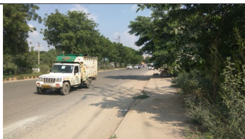
Poor mangement of pedestrian footpaths
