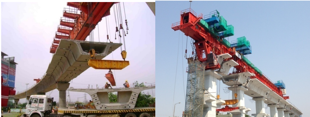
FIGURE 5.27: LAUNCHING OF BOX GIRDER SEGMENTS
