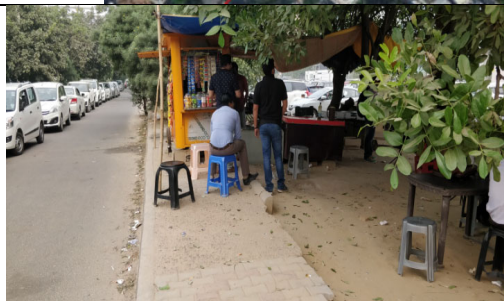
1. Encroachment of footpaths by vendors obstruct pedestrian movement
