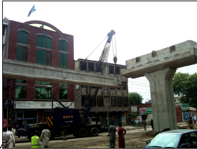
FIGURE 5.30: LAUNCHING OF I-GIRDER
