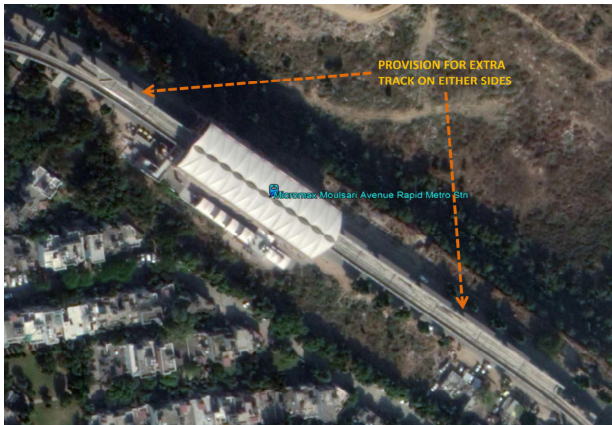
FIGURE 5.12: MICROMAX MOULSARI AVENUE RAPID METRO STATION
